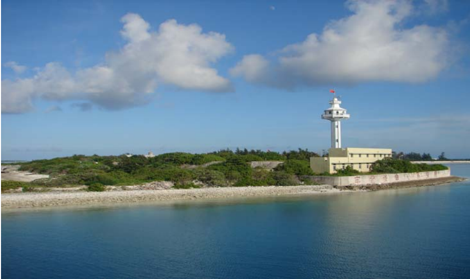
Duncan, Communication Tower
